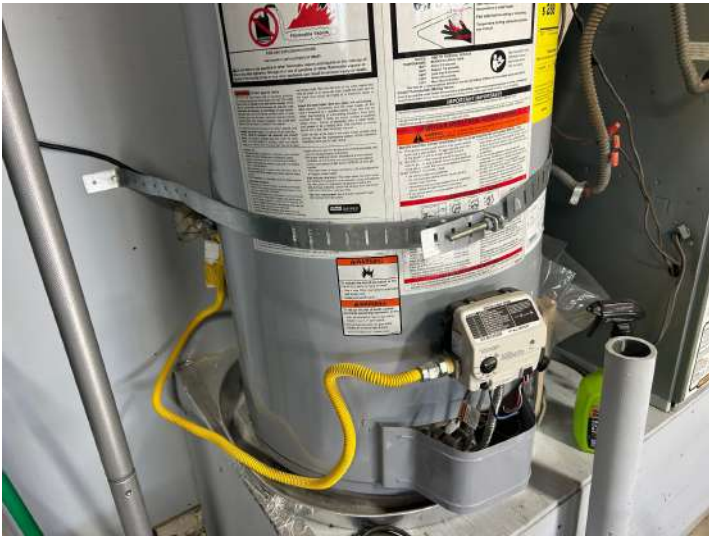
Photo 6.3A - Water heater — energy source, venting, TPR valve, seismic bracing
