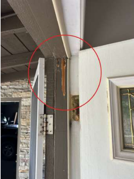
Photo 2.4A - All exterior doors
