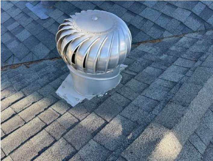
Photo 1.3A - Vents, flashing, skylights, chimney & penetrations
