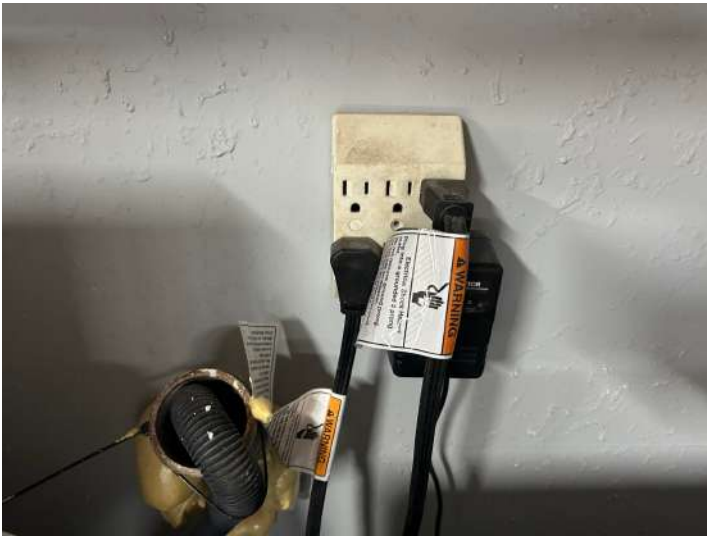
Photo 7.14A - Receptacle deficiencies
