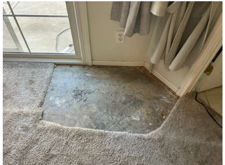
Photo 10.3B - Floors, walls & ceilings
